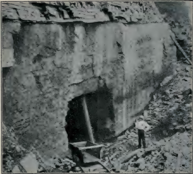
RUFFNER IRON MINE, ALABAMA Showing entrance to mine where ore beds are exposed
